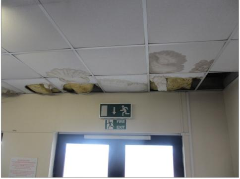
Figure 2: Evidence of water entering terminal building
