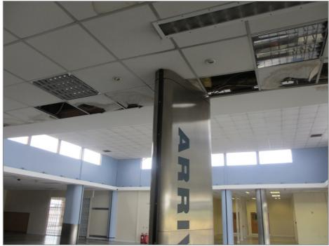
Figure 4: Evidence of water damage in may foyer.
