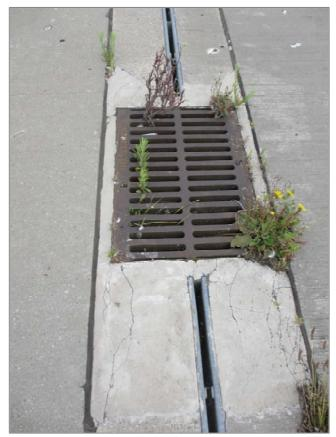
Figure 7: Apron Drainage. Some growth of plants which will need to be addressed.
