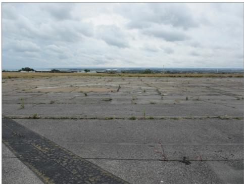
Figure 10: Shoulders of runway are paved. Evidence of plants establishing a presence in cracks
