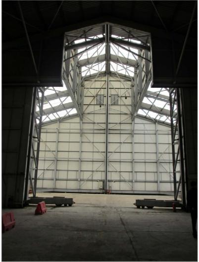
Figure 16: Bespoke tail enclosure of hangar
