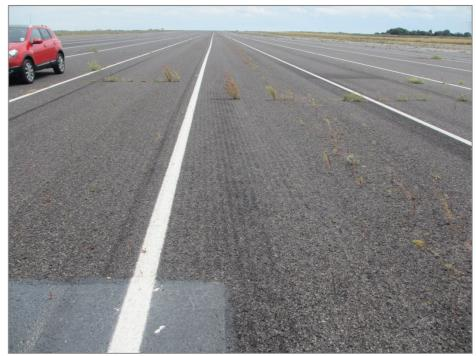
Figure 11: Runway 27 and evidence of plants establishing presence in cracks
